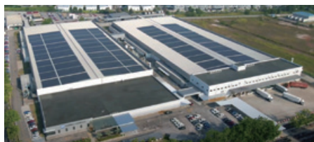
Photovoltaic power generation system (installation area of 17,059 square meters, power generation capacity of 3.4 MW) at the production facility
